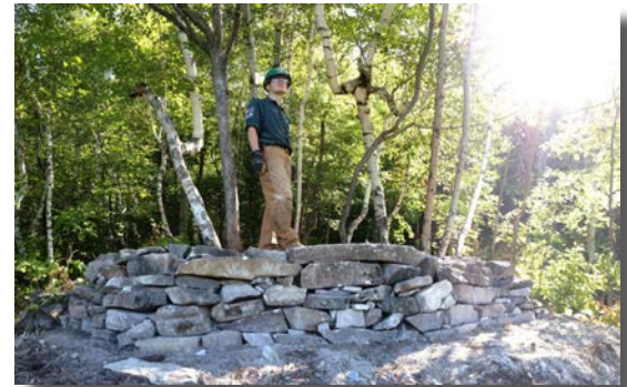
Admiring the work of the Dorset crew, atop a newly constructed retaining wall at Owl's Head Town Forest.
